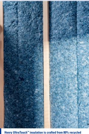
Henry UltraTouch<sup>™</sup> insulation is crafted from 80% recycled denim, lowering environmental impact and streamlining installation time without compromising performance
